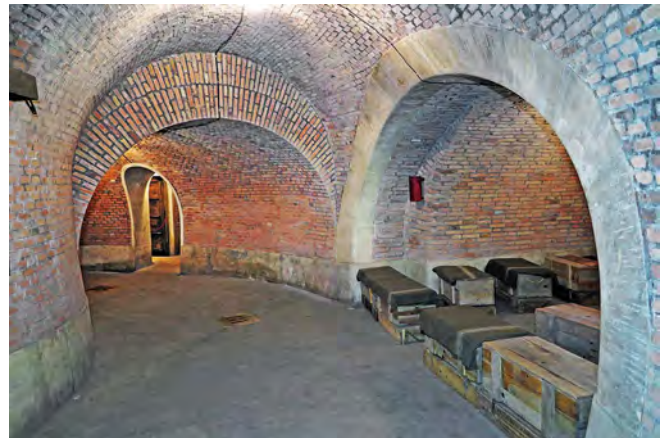
The turning area (on the right) for the Royal car in the Villa Ada shelter. The seating is modern and for visiting groups. The fine brickwork was heavily graffitied and has now been restored
